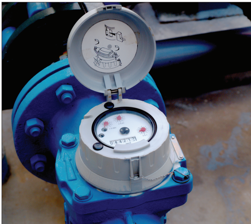
Water meters should be tested to protect customers against inaccuracies that could result in overcharges from overregistration and to protect water utilities from revenue losses resulting from underregistration. Photograph: krungchingpixs/Shutterstock
